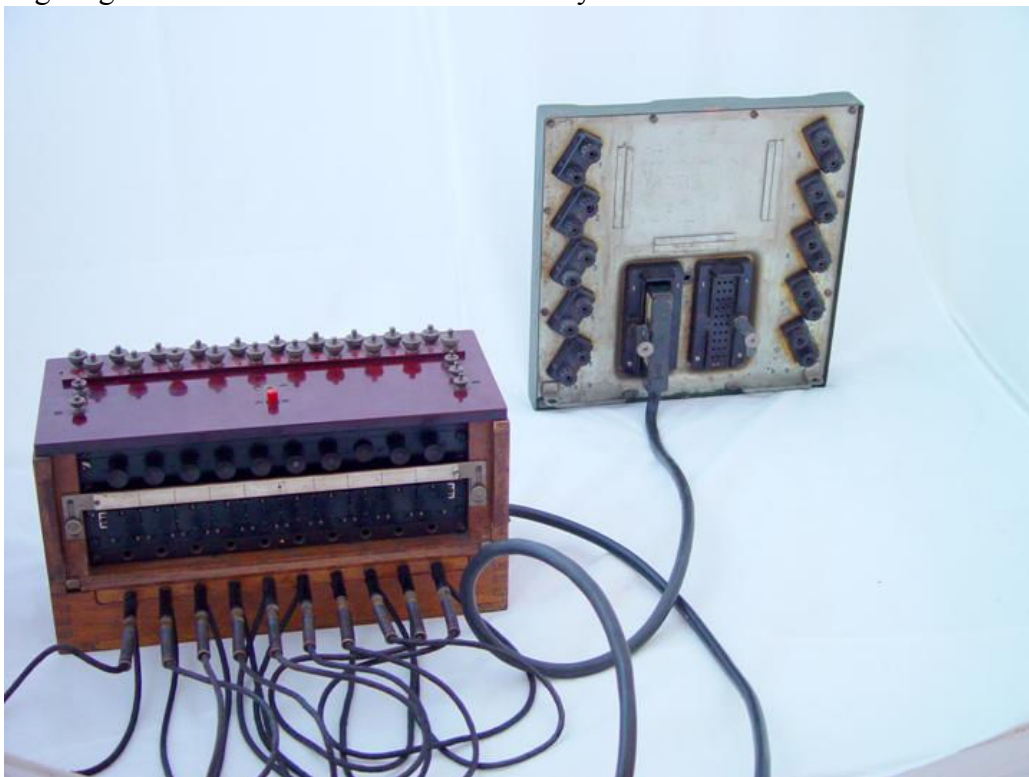
Figure 127: Remote line connection panel
